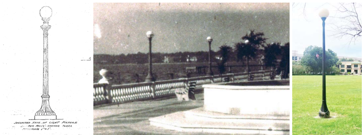
From left to right: light style suggested by Olmsted Brothers; lights as installed on the balustrade, c. 1925; current fixture with simple faceted (as opposed to more classical fluted) pole.
