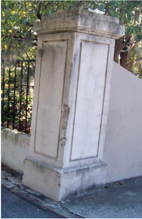
Northeast entry (left to right): damaged pier; peeling paint; damaged pier.
