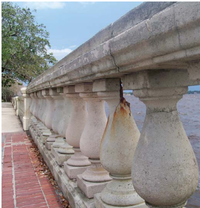
Above, original design detail of balustrade (courtesy Olmsted NHS) and circa 1949 appearance (courtesy JHS); below, current profile with added cap layer. Note also exposed, rusting reinforcing steel.
