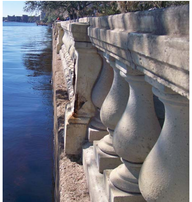
Above, original design detail of balustrade (courtesy Olmsted NHS) and circa 1949 appearance (courtesy JHS); below, current profile with added cap layer. Note also exposed, rusting reinforcing steel.
